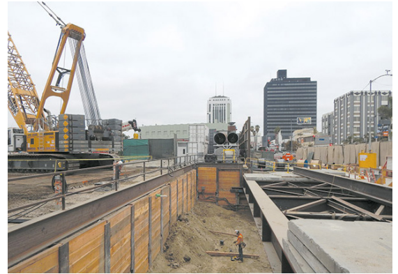
Coordination of underground utilities is critical to safely and efficiently operate Metro service.
