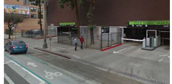
Driveways in close proximity to each other compromise safety for those walking to/from transit and increase the potential for vehicle-pedestrian conflicts.
